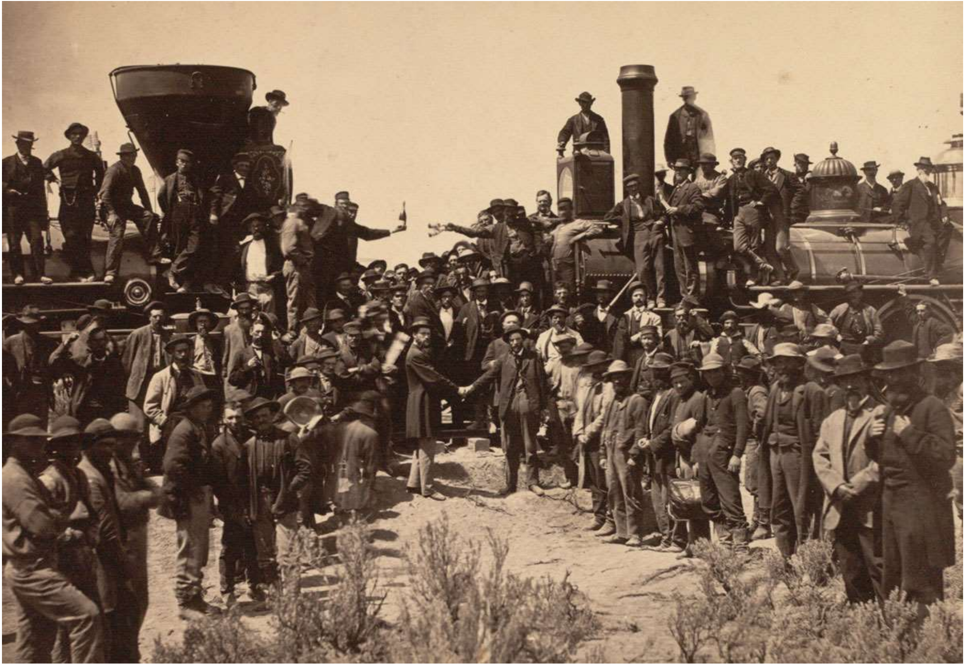
...to rails across the continent: infrastructure enabling influx and reinvention.
